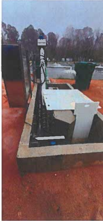
Photo 1: Archimedes screw screen
